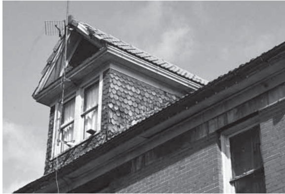
Original roofing and siding materials provide texture and visual interest.
