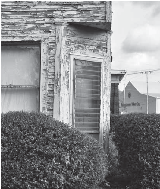
Remove peeling paint by scraping and sanding; never sandblast wood or masonry surfaces.
