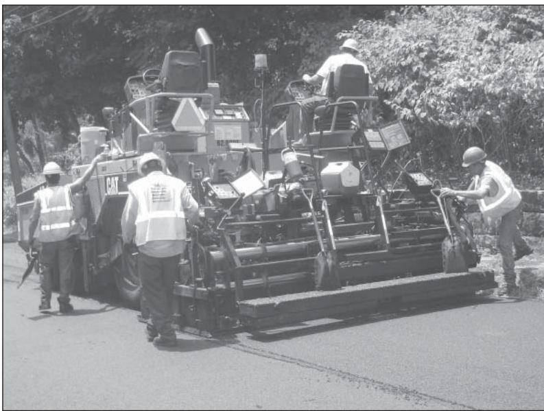
Crews repaved Walnut Street on July 30.
