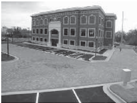
Permeable parking surface
