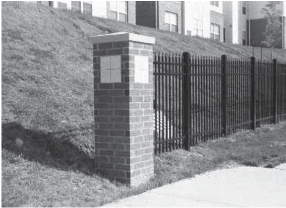
Parking lot fences should be appropriate to an urban setting
