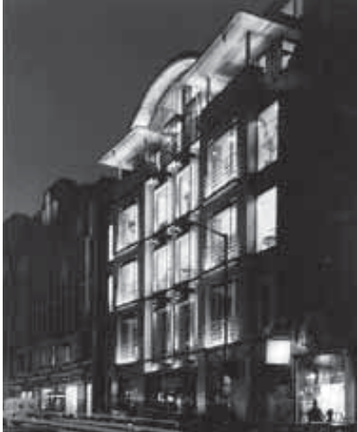
Exterior lighting draws attention to architectural features
