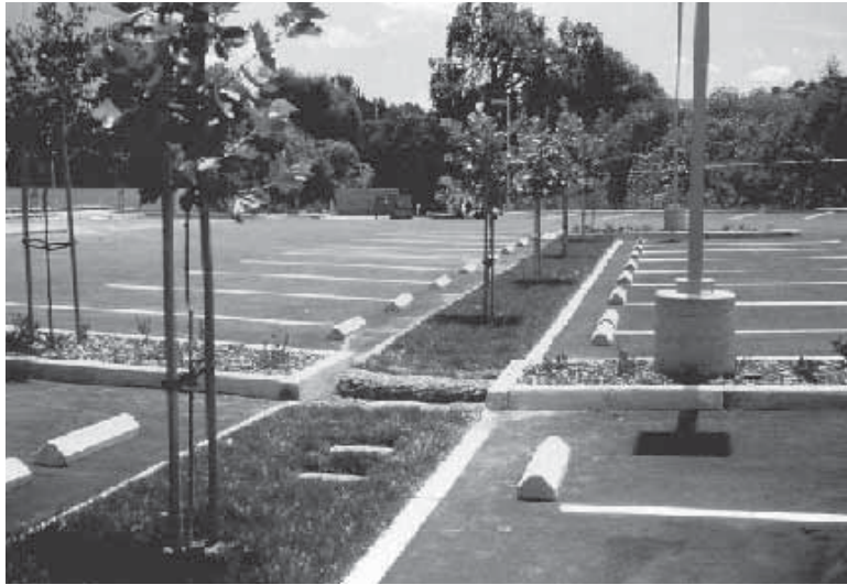
Vegetated swales in parking lots help to filter stormwater runoff
