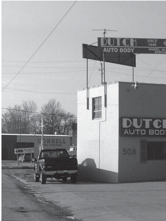
Wall and rooftop signs with a consistent typeface and design
